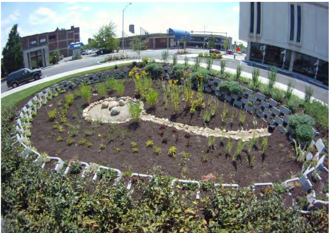
Figure 6: Photo of Typical Bioretention Basin
